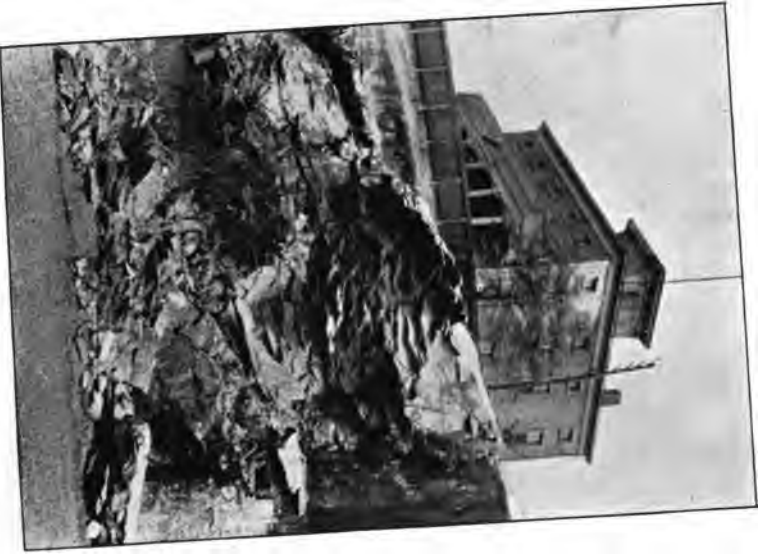
Fig. 1. Concentric jointing in diabase, Pa. R. R. cut, Jersey City. (Orphans Home, beyond, is built of diabase.)
